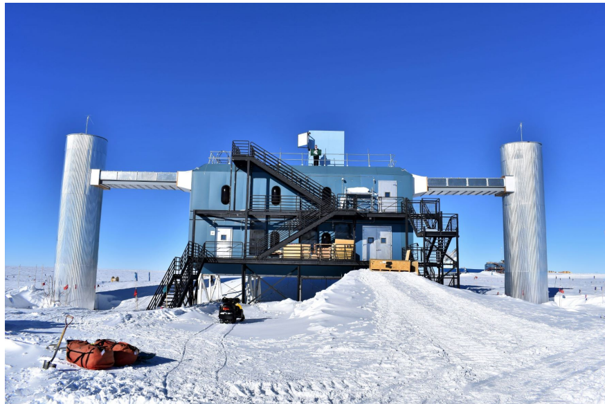
Figure 3.4: An image of the IceCube Laboratory (ICL) on the surface above IceCube. The ICL is the main operations building on-site at the South Pole, with laboratory working space on the first floor and the server room on the second floor. The cables from IceCube are routed along the surface to the two cable towers on each side of the ICL, which are both connected to the server room on the second floor.
