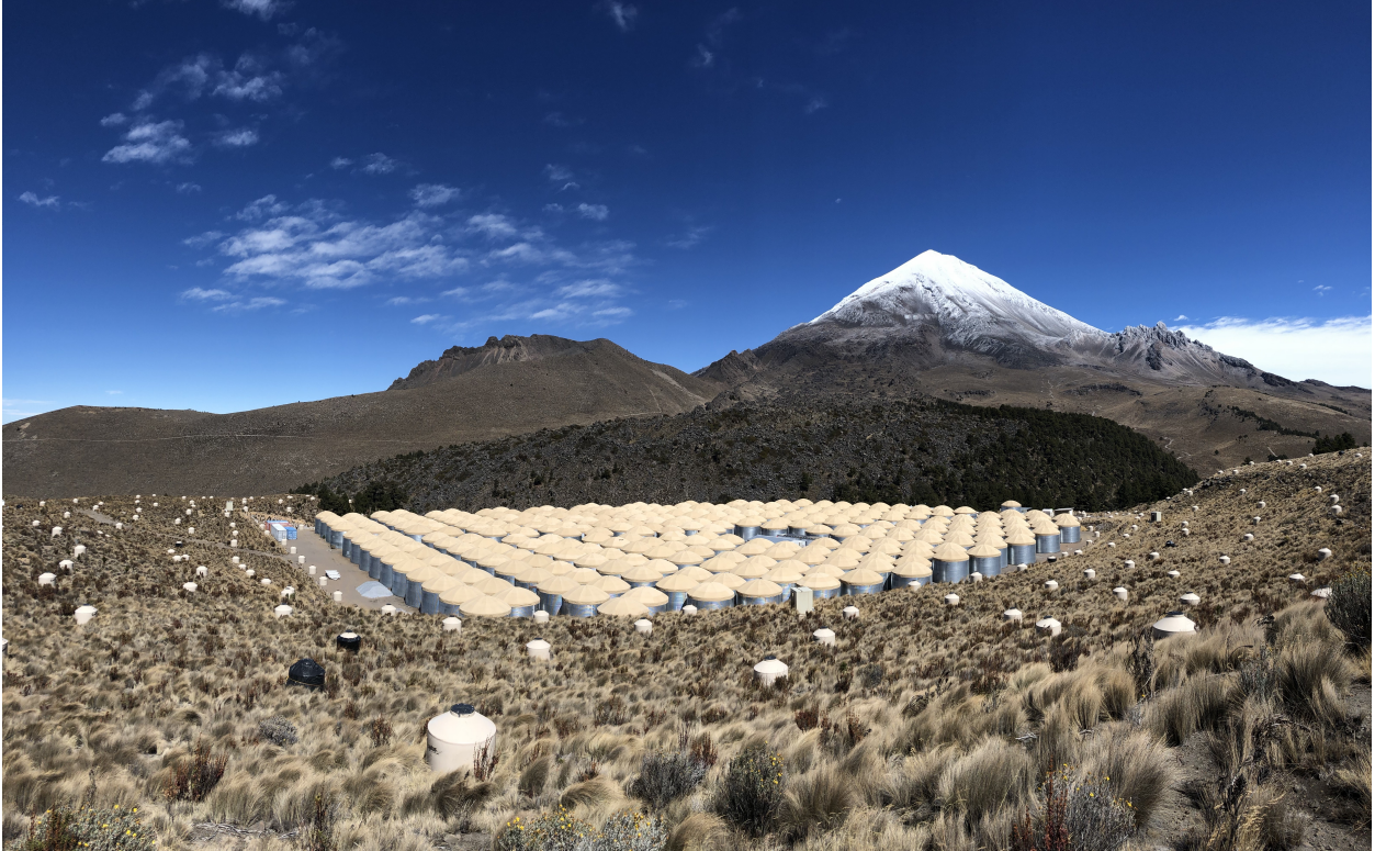
Figure 2.1: A photograph of the HAWC detector showing the main array and the surrounding outrigger tanks taken in February 2020. The mountain Pico de Orizaba can be seen in the background.
