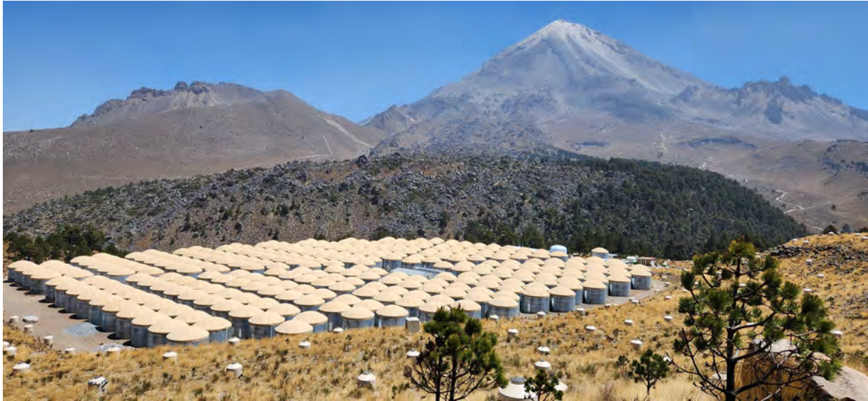
Figure 2.1 The HAWC Observatory circa April 2024. The main array is a concentration of large tanks, with the outrigger array containing the much smaller tanks seen on the surrounding hillside. The mountain Pico de Orizaba is visible in the background. Photo taken by myself.
