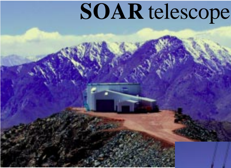
Last September as construction began on the dome
