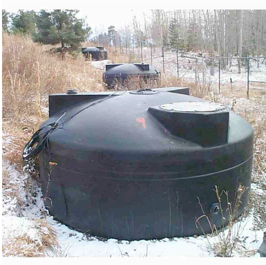
Figure 5.7: Photo of an outrigger tank.
